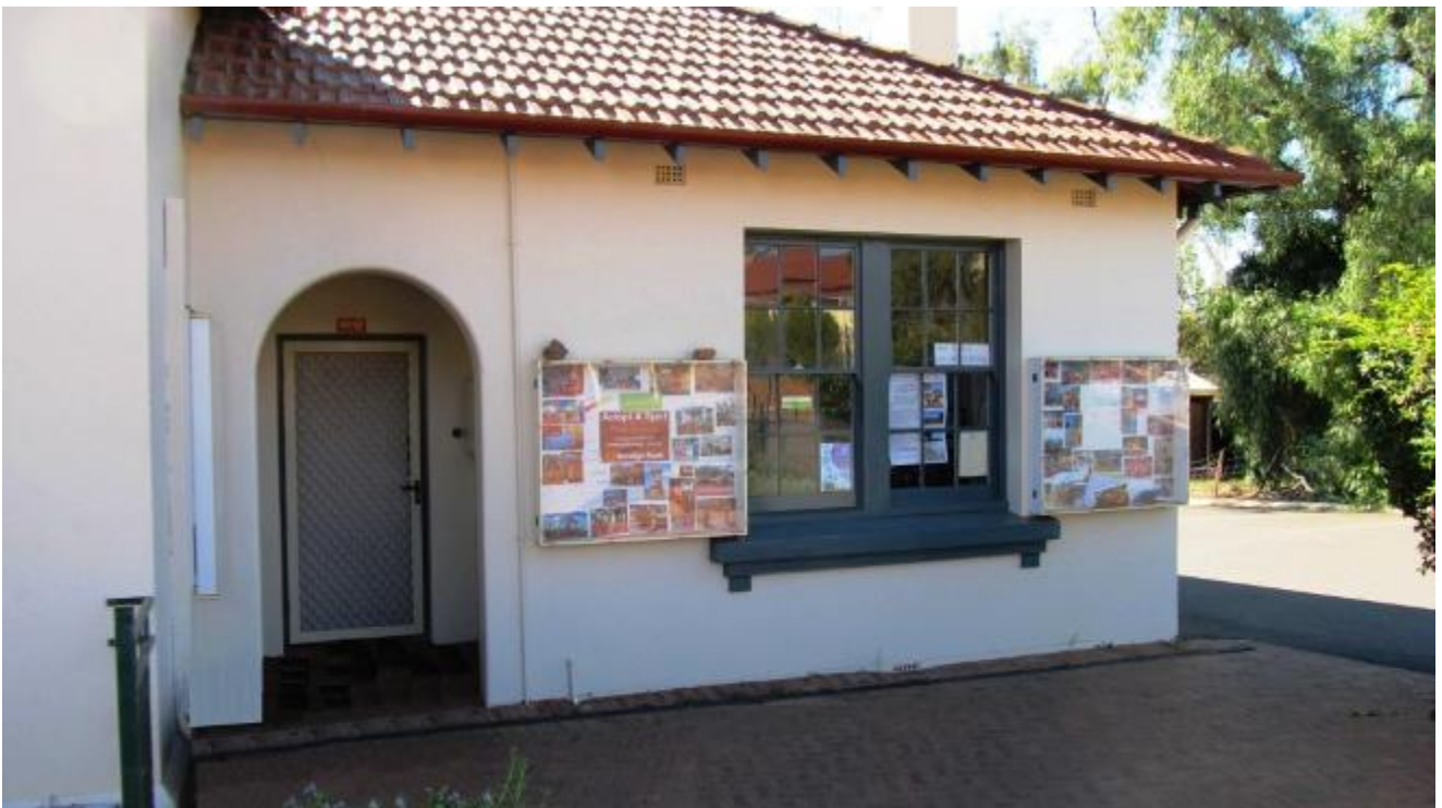
Above: Drummond House Stirling Terrace entry
